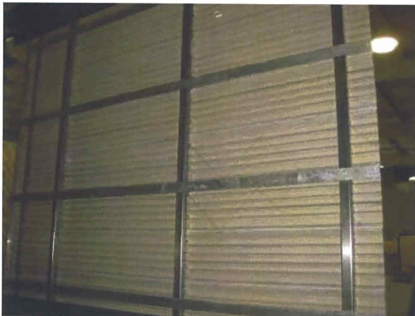
Photo No. 2 Interior Framework of the NeaCera ® Terra-cotta Rainscreen Cladding System
