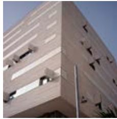
Los Molinos Building | Tenerife | Spain
