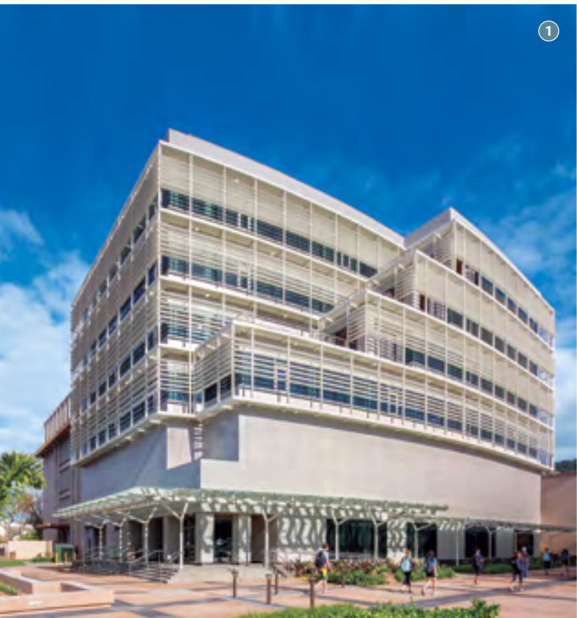
1 University of Hawaii Information Technology Center, Cantilevered Sunshades Architect: Ferraro, Choi and Associates
