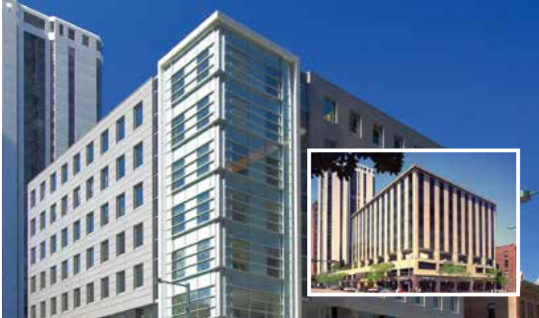
Larimer Office Complex | Denver, CO
