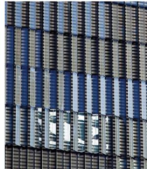
On the building's lower floors, a blast-resistant grille is sandwiched between open glass panels and the louvers, providing its base with security and breathability.
