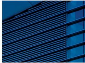
Architectural firm Integrated Design Solutions chose Construction Specialties RS-7315 Storm Resistant Louver for the exterior of the 220,000 sq. ft. George G. Brown Memorial Laboratories building at the University of Michigan because of its high airflow, excellent water resistance and two-piece blade design.
