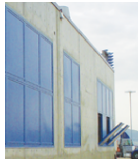
Bottom hinged Explovent panels were field tested during the installation process.
