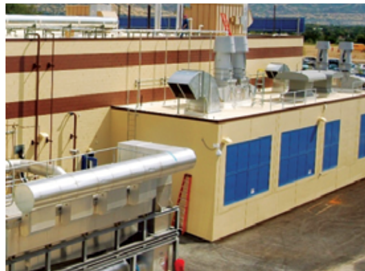
Ethylene gas is used to sterilize medical equipment in this facility's storage building. Explovent panels were specified to release pressure build-up from the gas if ever necessary.
