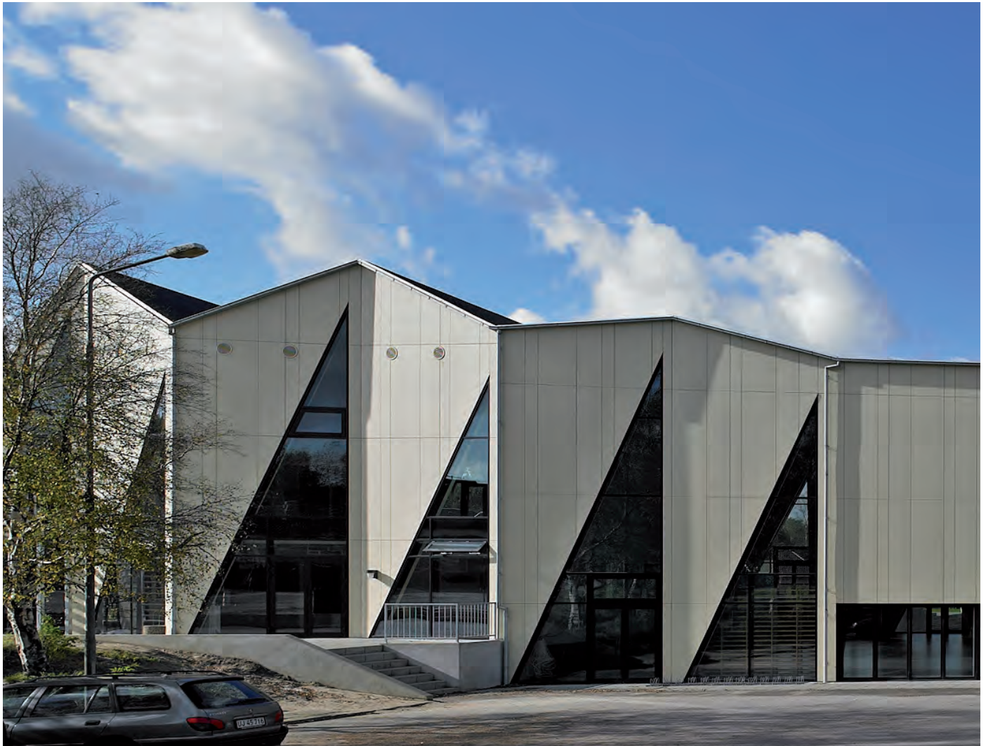
DENMARK Sports Hall Kibaek Krydsfelt, Kibaek
