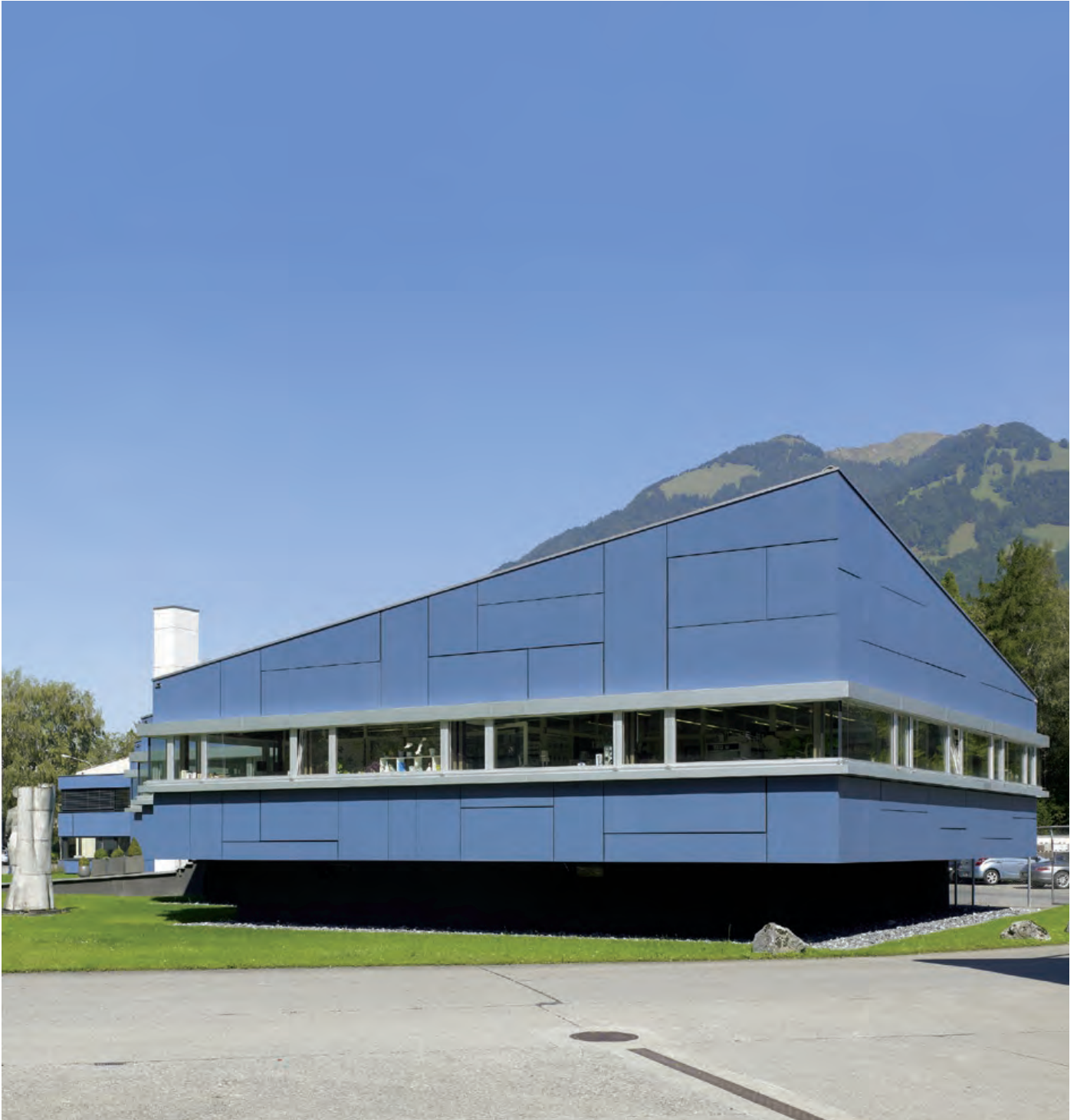
SWITZERLAND Office Building, Niederurnen
