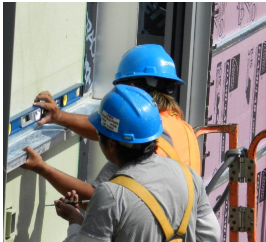
Figure 3.2a (Initial Sub-construction Installation)
