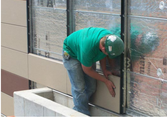
Figure 6.1 (Executing the Lift & Lock System)
