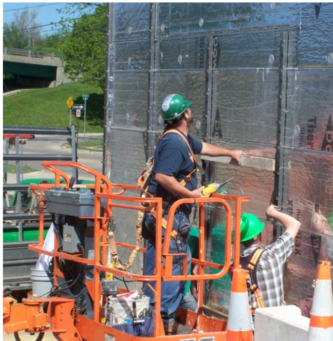
Figure 5.2 (Installing Support Profile Using a Spacer)
