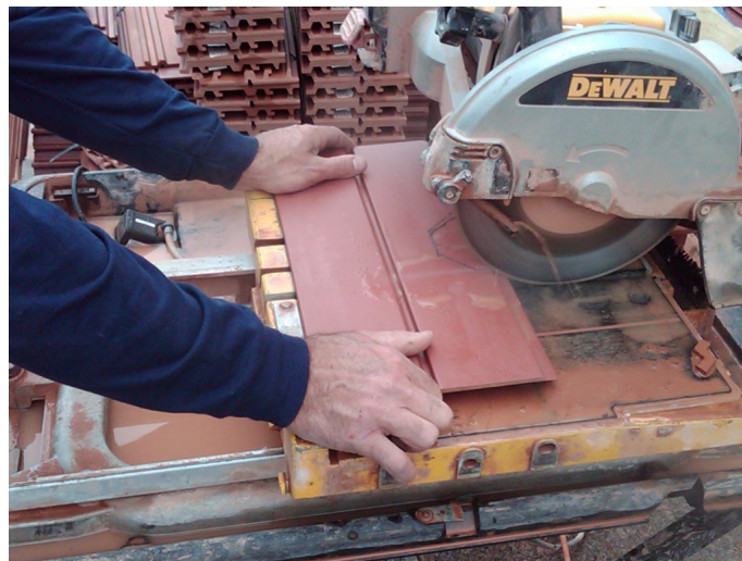
Figure 6.2 (Cutting NeaCera® Panels)
