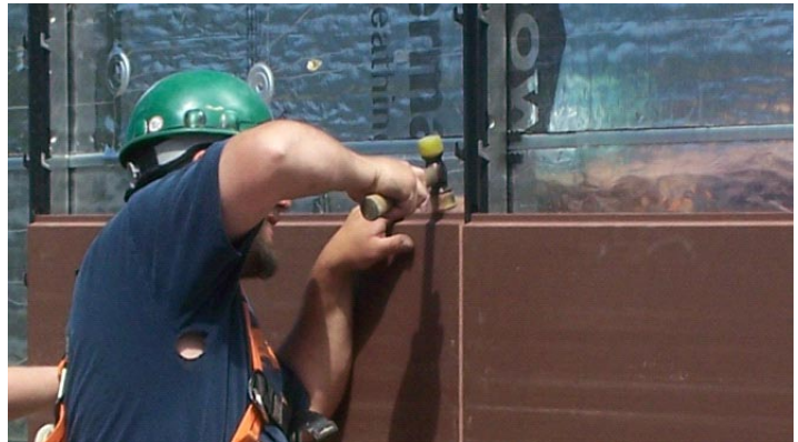
Figure 6.1 (Executing the Lift & Lock System)
