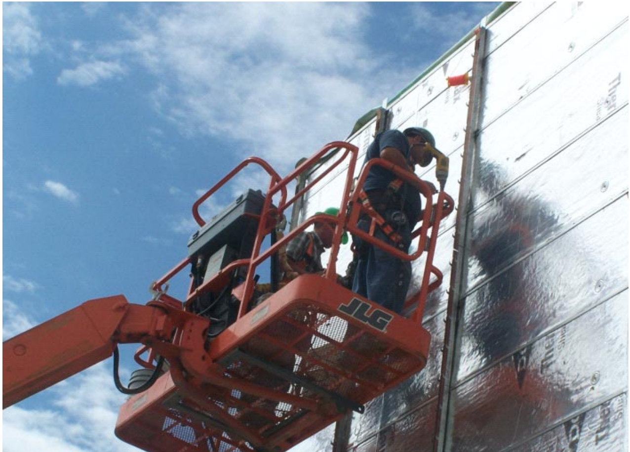
Figure 5.1b (Installing the Initial Support Profile)
