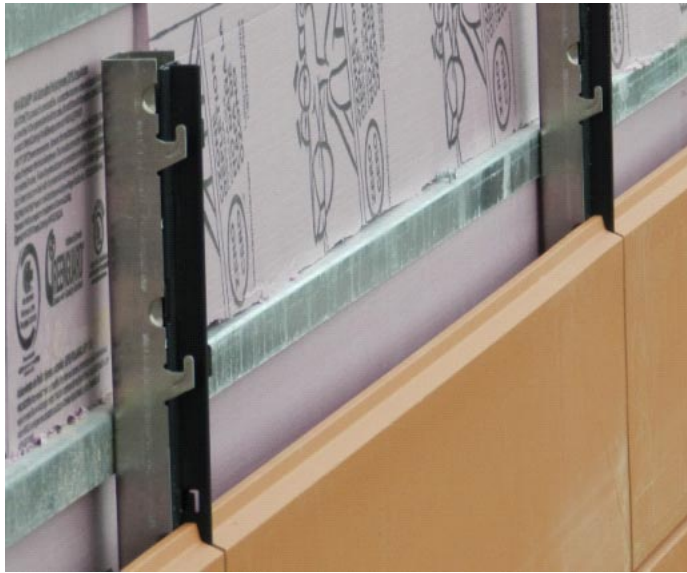
Figure 5.3 (Support Profiles with Joint Inserts)
