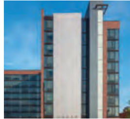
Page 34 Westin Hotel Birmingham, AL A: Rabun Architects C: Brasfield & Gorrie D: National Panel Systems
