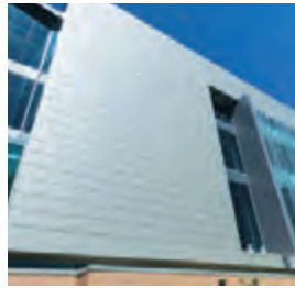
Page 14 Erie County Medical Center Buffalo, NY A: IKM, Inc. Architects and Kideney Architects C: LP Ciminelli D: Arrow Sheet Metal Works, Inc.
