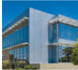
Page 26 Regional Transportation Management Center New Orleans, LA A: Sizeler Thompson Brown Architects C: The Shaw Group, Inc. D: F.L. Crane and Sons
