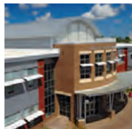
Page 42 Renaissance Academy Virginia Beach, VA A: RRMM Design Build C: W.M. Jordan Company D: Metal Crafters, Inc.
