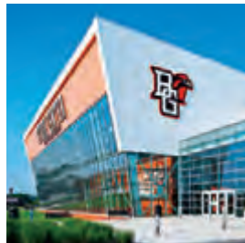
Page 18 Stroh Center Bowling Green, OH A: Rossetti C: Mosser Construction D: Crown Corr, Inc.
