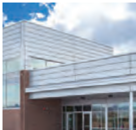
Page 31 Neil Armstrong Academy West Valley, UT A: Naylor Wentworth Lund Architects C: Darrell Anderson Construction D: Steel Encounters, Inc.
