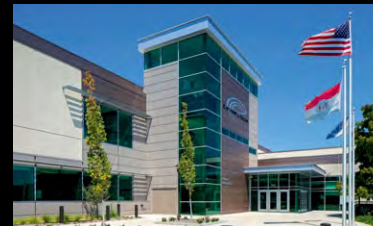
Page 39 Buescher Hall East Central College Union, MO A: The Lawrence Group C: K&S Associates, Inc
