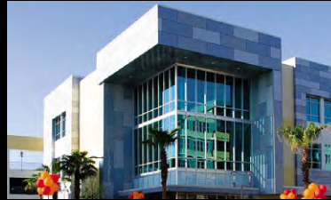
Page 25 SODO Orlando, FL A: Cupkovic Architecture, LLC C: Hoar Construction, LLC
