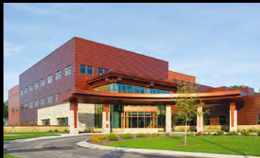
Page 34 North Memorial Hospital Medical Office Building Maple Grove, MN A: BWBR Architects C: D. J. Kranz Co., Inc.
