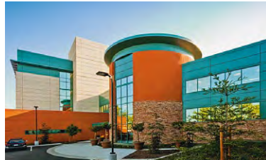
Page 9 Lodi Memorial Hospital Lodi, CA A: HDR Inc. C: Harbison-Mahony-Higgins Builders Inc.
