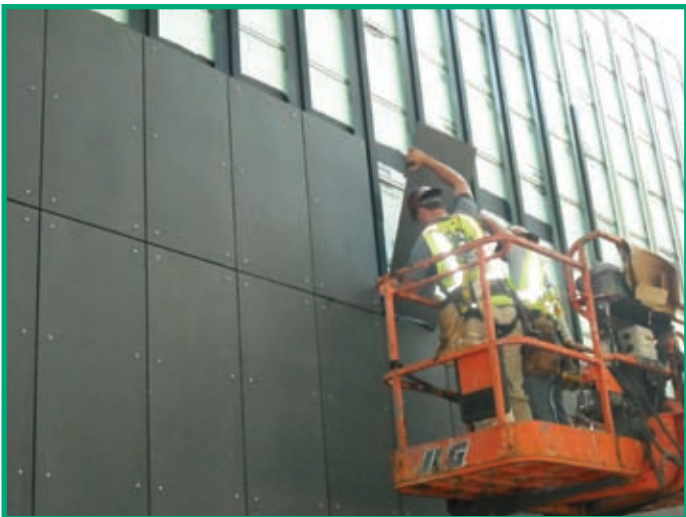
Tony Strickland's crew installing Fibre C panels at the UGA Butts-Mehre Expansion
